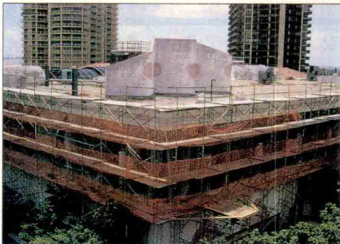
Completed: The roof slab was raised 11 ft, very slowly, over 26 days.
