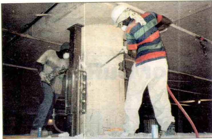
Workers chipped away at column concrete (left) to expose reinforcing steel (right) that was cut just before roof lift began.
