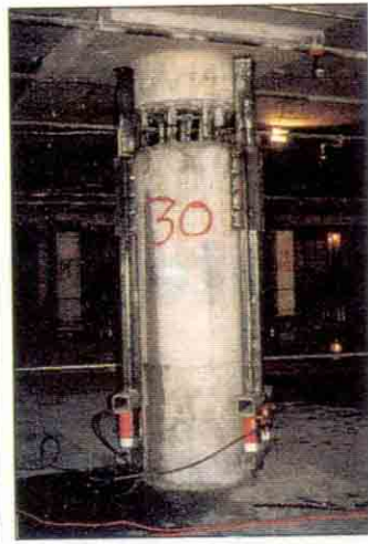
Workers chipped away at column concrete (left) to expose reinforcing steel (right) that was cut just before roof lift began.
