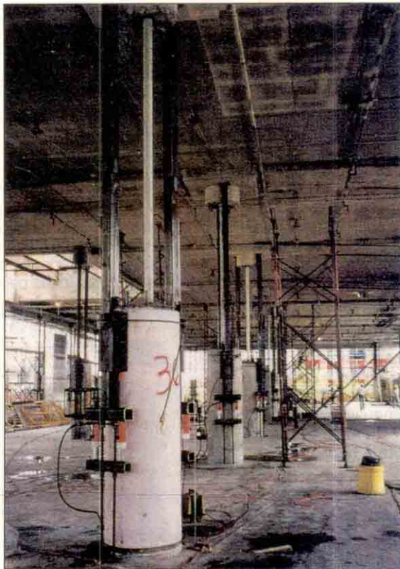
Columns were fitted with lifting mechanism, temporary posts.
